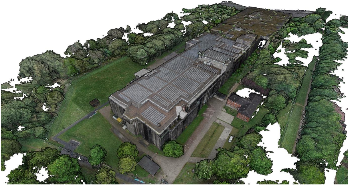
Fig 3. Final 3D model from the outside part of the Bunker, ready for visualization.
